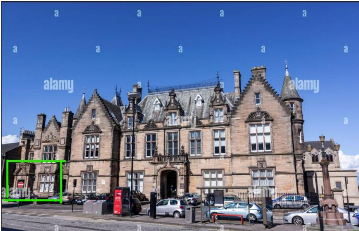
Front view of new premises, Viewfield Chambers
